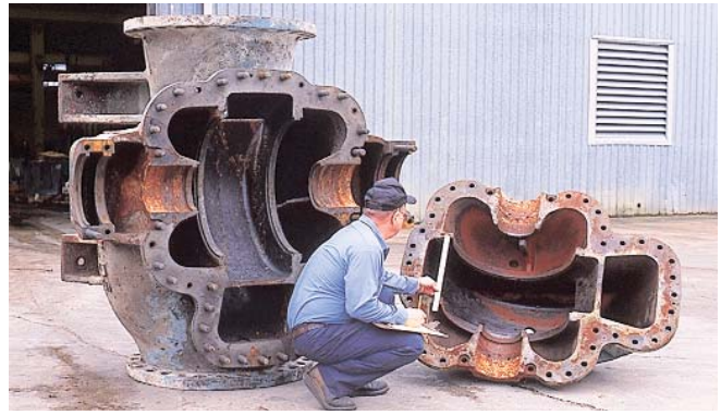
Disassembled pump is inspected for unusual wear.
